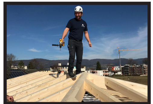
Assembly of prefabricated wooden elements
