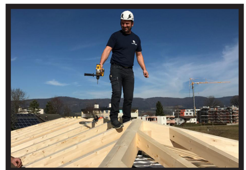
Assembly of prefabricated wooden elements
